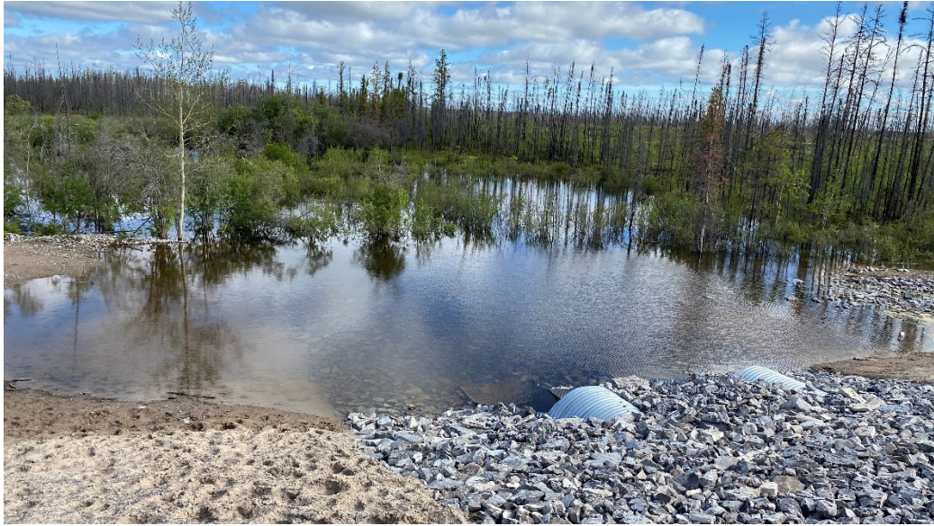
Figure 1. A small standing water area at one of the numerous culverts along the Tlicho Highway. Such waterbodies may be seasonally or annually ephemeral.
